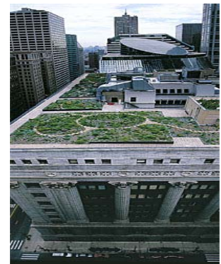
Figure 14—Chicago, Illinois, requires most major buildings to have green roofs.
