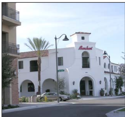
Figure 45— The ground floor of mixed-use buildings should be highlighted through the use of arcades, prominent entries, and other similar features.
