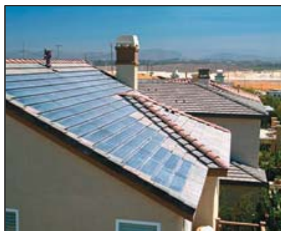
Figure 11—Proper solar orientation of a residential structure or lot can help maximize the efficiency of solar panels and solar thermal heating devices.
